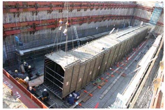
Installation of Neutrino Decay Volume
